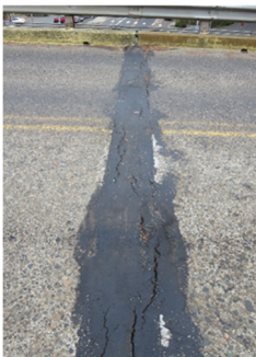
In-span deck joint, OR Approach
