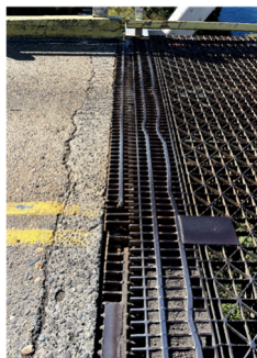
Truss deck joint at OR Approach
