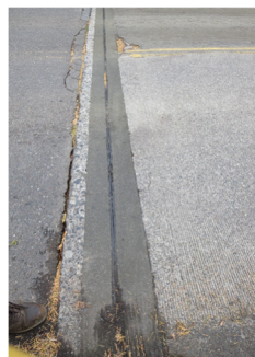
WA abutment deck joint
